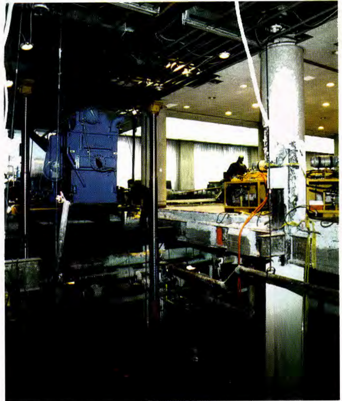
An alert building manager replaced this midtown structure's aging chillers as soon as a first floor retail bank lease expired. In this picture the two-stage chiller is about to be lowered into the basement using hydraulic jacks.
