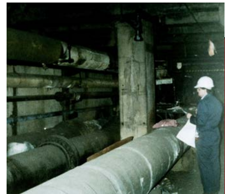
Inspecting the utility tunnels
