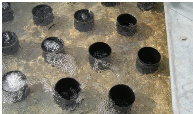
Photo 1: Adding cup extensions to the center pan orifices maximizes contact during low flow at the tower perimeter.
